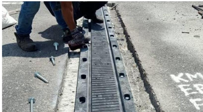
The joint is allowed to cool to ambient temperature and may be trafficked in 1 – 2 hours.
